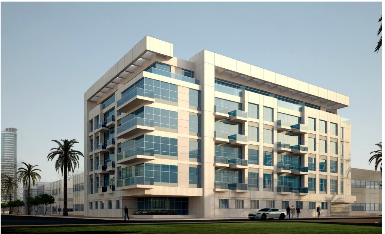
(B+G +5 Typ + R) Residential Building on Plot No: IC3-F-12 For Mr. Isam Abdul Rehman Bayasin Al Amoudi International City, Dubai UAE
