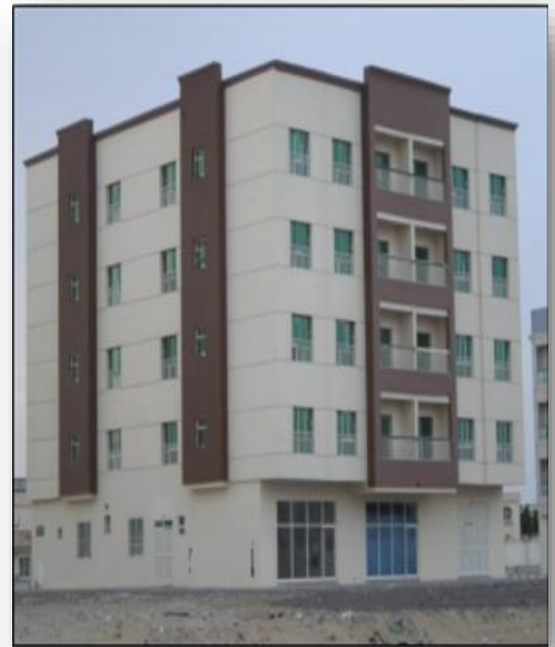
(G + 4) Residential Building For Mr. Abdel Kader Amer Ghawey Al Jurf, Ajman UAE
