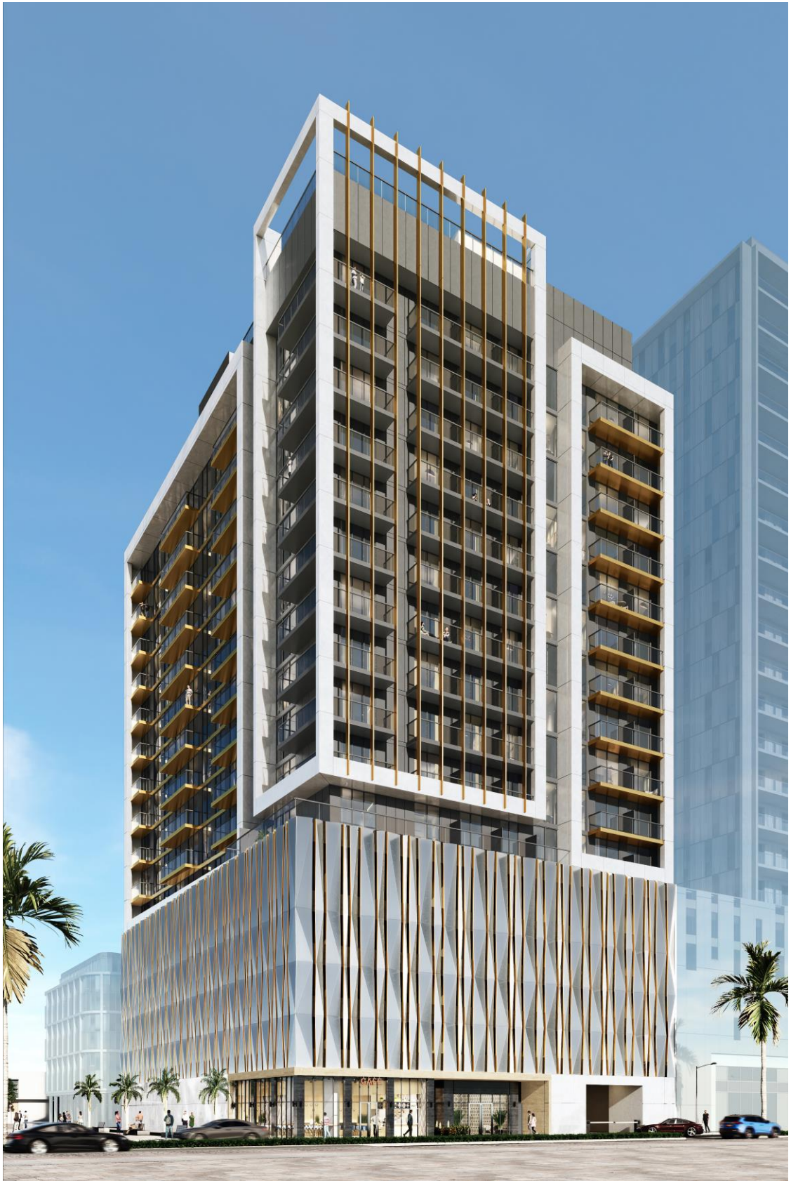
(G + 4P+11+R) Residential Building On Plot No: JVC16MRM002 For Circle Capital Investments FZCO JVC, Dubai UAE
