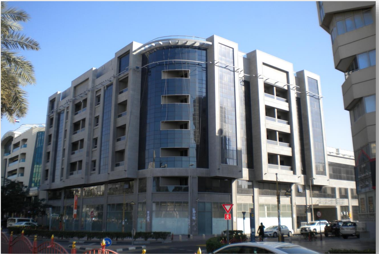
(2B + G + 4 Type) Hotel Building For The Bristol Inn / Gulf Inn Hotel Al Muteena, Dubai UAE
