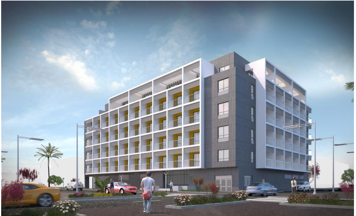
(B+G+5) Residential Building on Plot No: IC3-F-52 For Mr. Adnan Ahmed Hamdan Ahmed Abuomar International City, Warsan-4th, Dubai UAE
