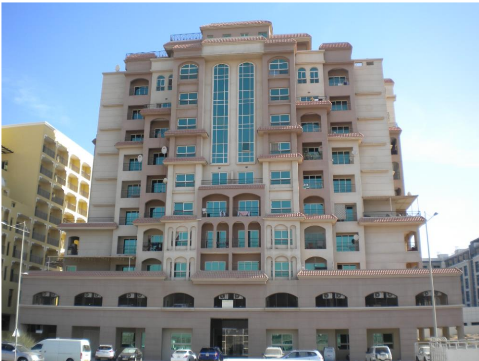
(G + P +8 Typ + R) Residential Building on Plot No: H39 For Mr. Abdul Jalil Al Asmawi International City, Dubai UAE
