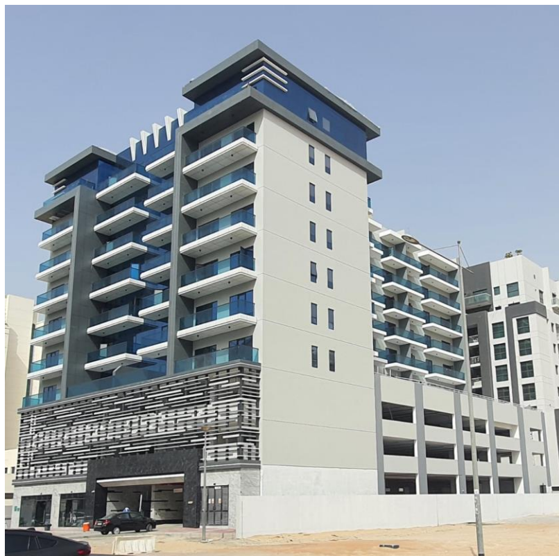
(G + 2P +7) Residential Building on Plot No: IC3-L-11 For Mr. Kamil Hashim Mohammed Essarohe International City, Warsan-4th, Dubai UAE
