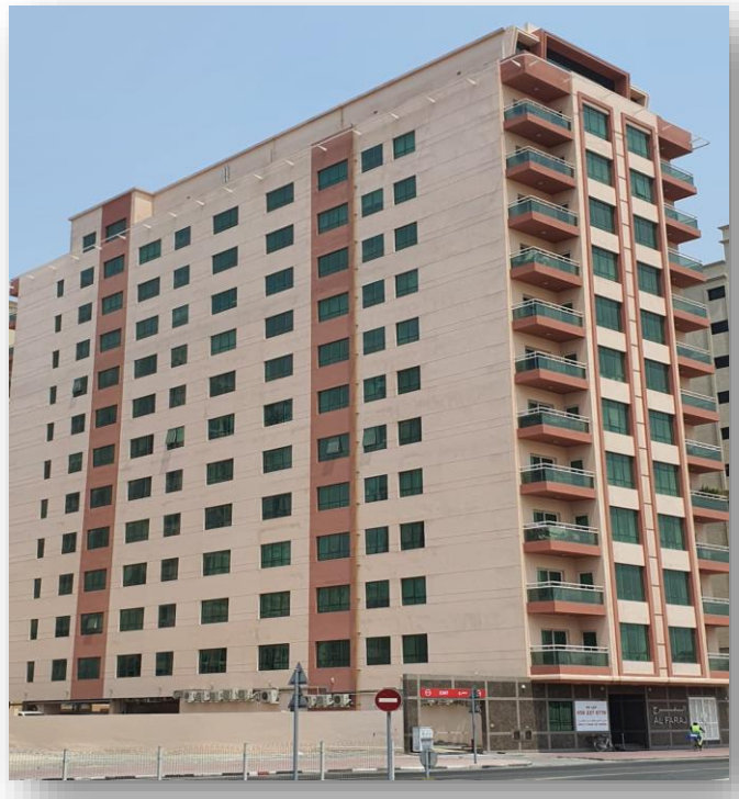
(B + G + 11) Residential Building For Mr. Faraj Amrulla Abdulla Abdul Rahim Al Nahda 2 nd , Dubai UAE
