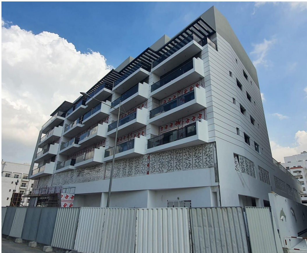
(G + P + 4) Residential Building on Plot No: IC3-G-12 For Mr. Khaled Abdul Kader Karimeh International City, Warsan-4th, Dubai UAE
