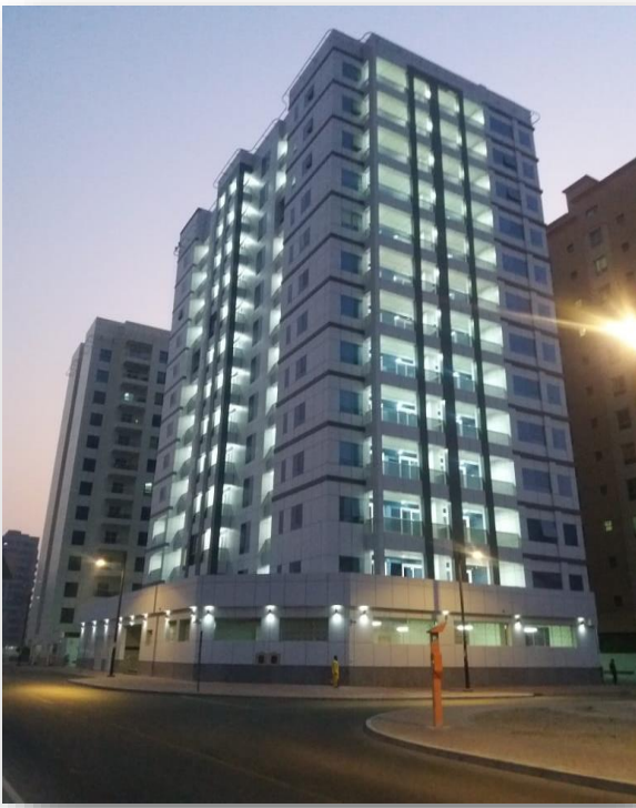
(B + G +12 + HC ) Residential Building For Mr. Rashid Mohamed Mubarak Al Mansoor Al Nuami Al Nahda 2, Dubai UAE
