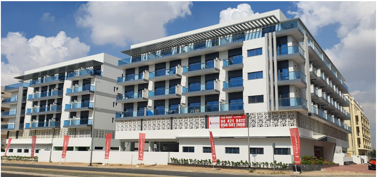
(G + P + 4) Residential Building - 2 Nos on Plot No: IC3-B-17 & IC3-B-22 For Mr. Khaled Abdul Kader Karimeh International City, Warsan-4th, Dubai UAE
